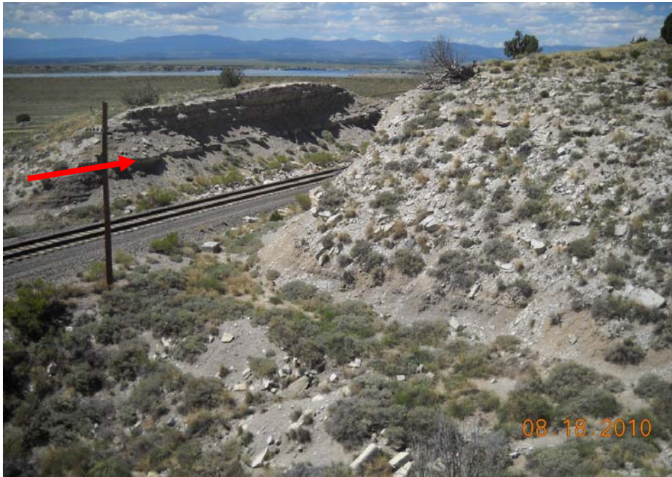
Photograph 7: Railroad cut through the interbedded limestone and claystone of the Greenhorn Limestone formation, near UPRR-1. The thicknesses of the limestone layers are between about 0.8 to 1.5 feet. The arrow points to a limestone layer.
