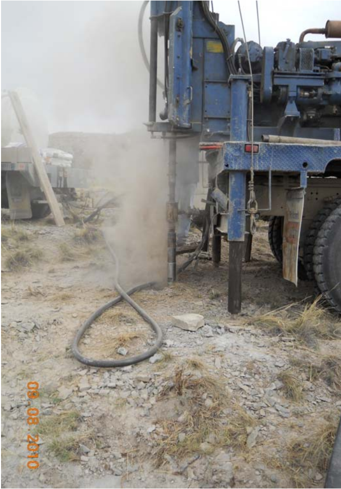
Photograph 8: Drilling with pressurized air and a down-hole hammer through the interbedded limestone and claystone.
