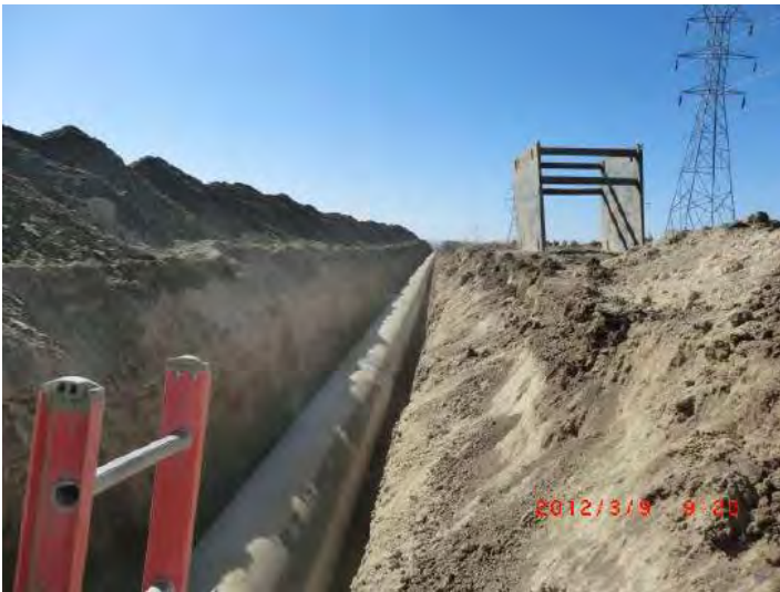
OPEN TRENCH EXCAVATION
