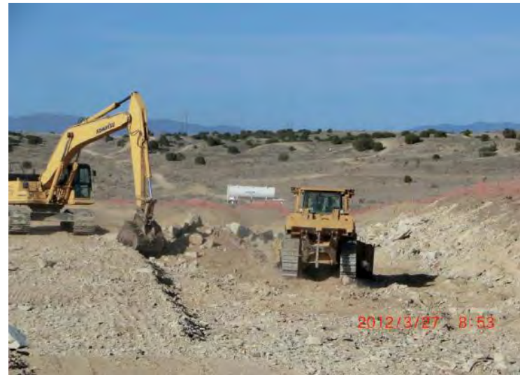
SUBCUTTING FOR ROCK TRENCHING OPERATION
