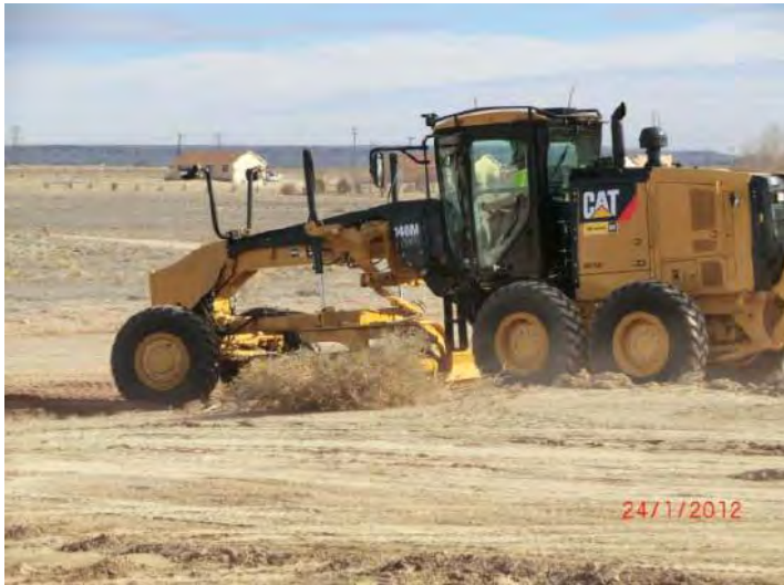
CREW CONSTRUCTING SOIL BERM FOR BMP
