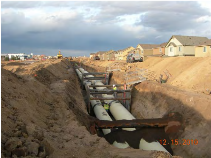
DUAL FINISHED WATER PIPE INSTALLATION
