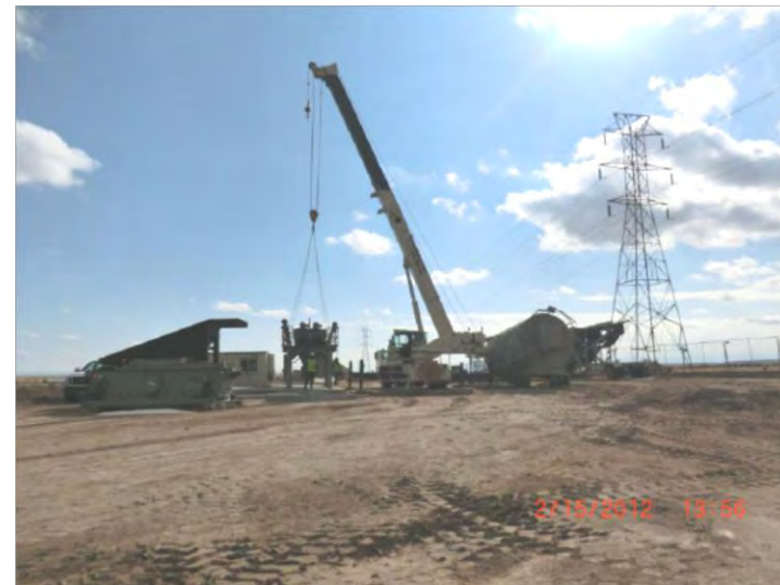
BATCH PLANT ASSEMBLY
