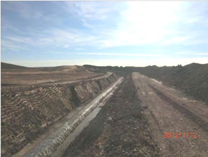
N1B CONTROLLED LOW-STRENGTH BACKFILL MATERIAL PLACEMENT
