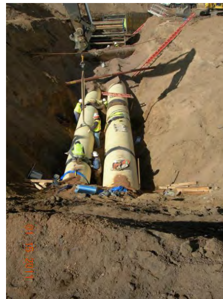
DUAL FINISHED WATER PIPE INSTALLATION
