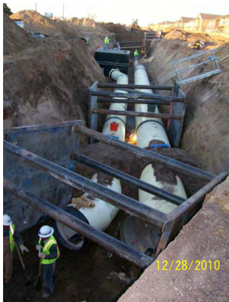
DUAL FINISHED WATER PIPE INSTALLATION
