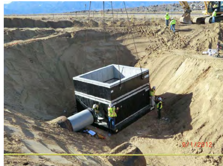
AIR VACUUM VAULT SECTION PLACED FOR 42" PIPELINE
