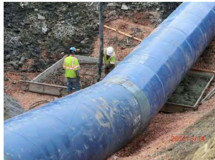
BLOWOFF FOUNDATION CONSTRUCTION
