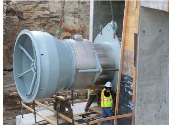
PLACING FIXED CONE VALVE
