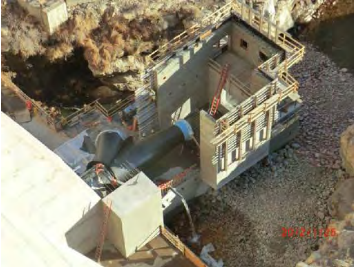
VIEW OF WYE SECTION AND VALVE FACILITY FROM TOP OF PUEBLO DAM
