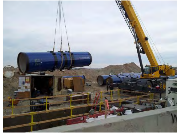
PIPE PLACEMENT FOR HIGHWAY 50 TUNNEL CROSSING
