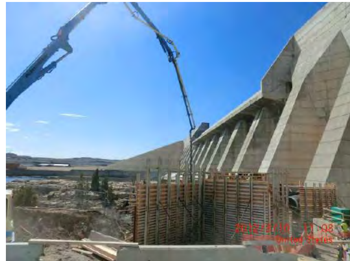
PUMPING CONCRETE AT NORTH SHORE RETAINING STRUCTURE
