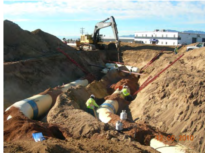
DUAL FINISHED WATER PIPE INSTALLATION
