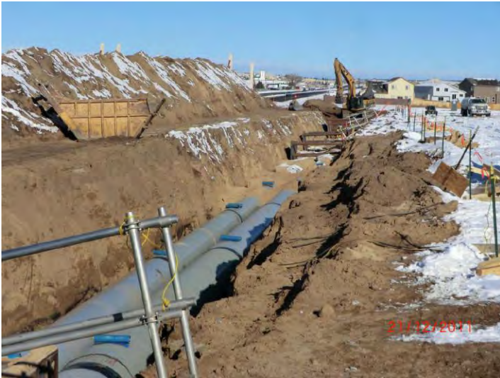
DUAL PIPE INSTALLATION IN COMMON TRENCH
