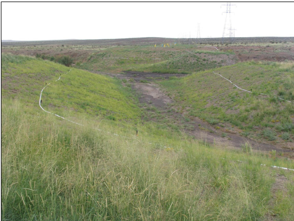
Photo 8. Vegetation growth on erosion control netting installed at the Steel Hollow Crossing point along the S3 section of the SDS pipeline (looking southeast). September 12, 2013.
