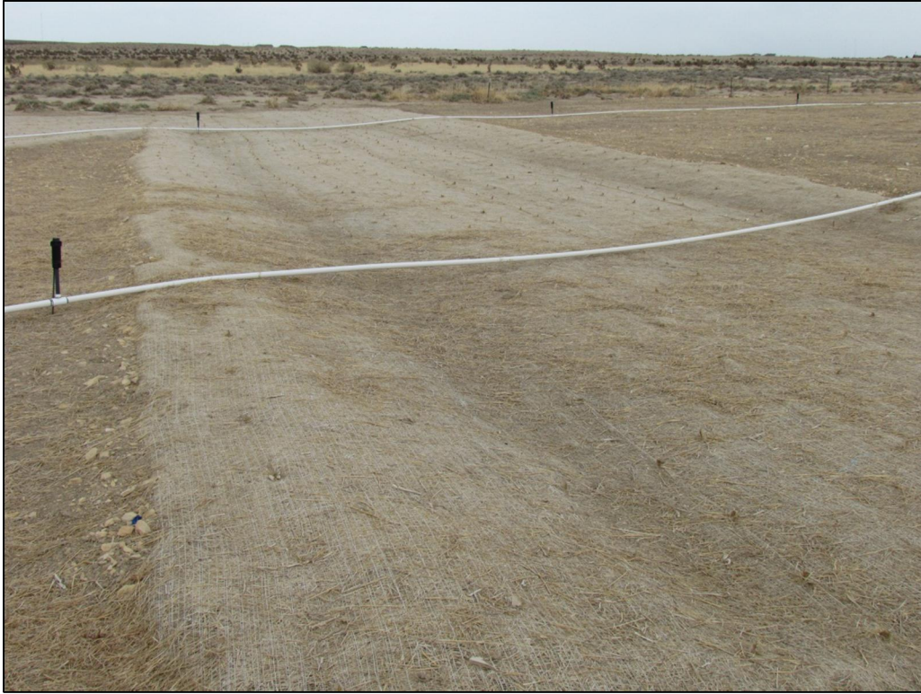
Photo 3. Small drainage with erosion control netting near Southern end of the S3 section of the SDS pipeline. April 30, 2013.
