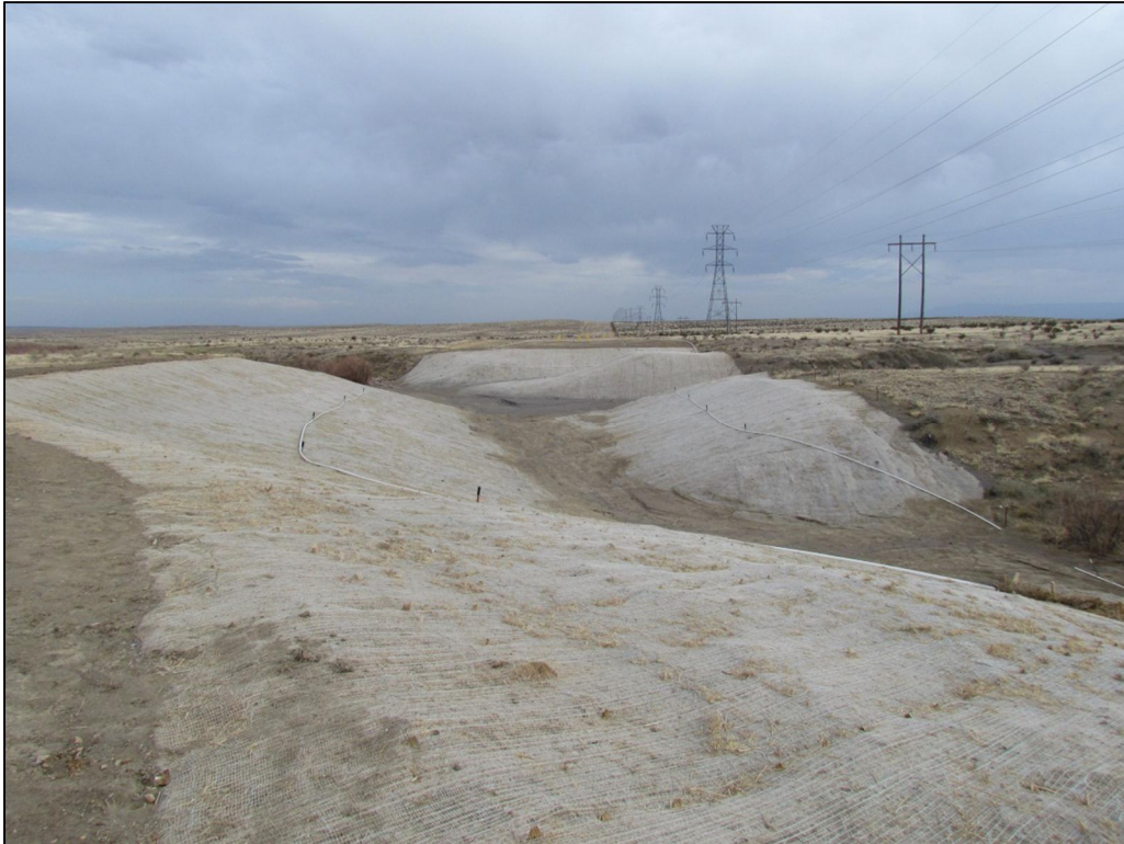
Photo 7. Erosion control netting installed at the Steel Hollow Crossing point along the S3 section of the SDS pipeline (looking southeast). April 30, 2013.
