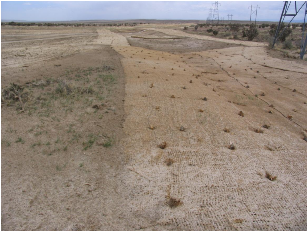
Photo 10. Drainage repair north of Steel Hollow S3 Section of the SDS Pipeline Route. Photo taken at N38° 28' 40.1"; W104° 41' 25.9", looking southeast. April 29, 2014.
