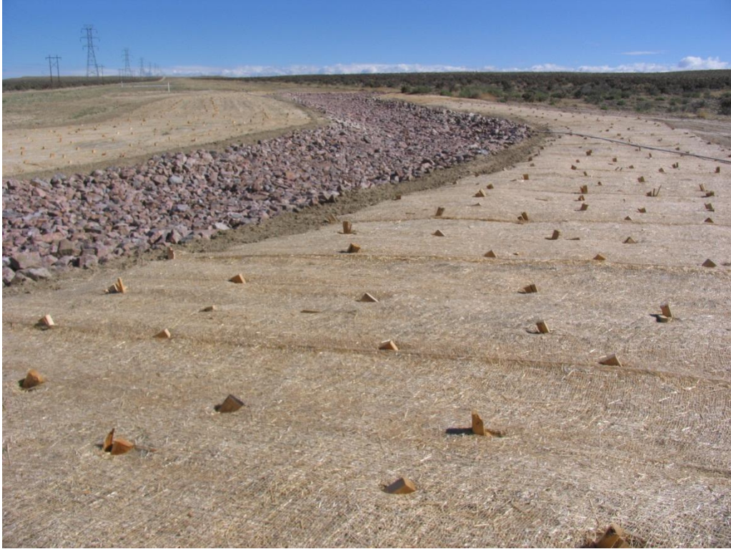
Photo 3. Installed rock rip-rap channel - S3 Section of the SDS Pipeline Route. Photo taken at N38° 26' 15.3"; W104° 41' 24.3", looking north. April 30, 2014.
