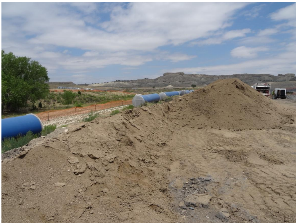
Photograph 4: Stockpiles from excavation on western side of site with no control measures
