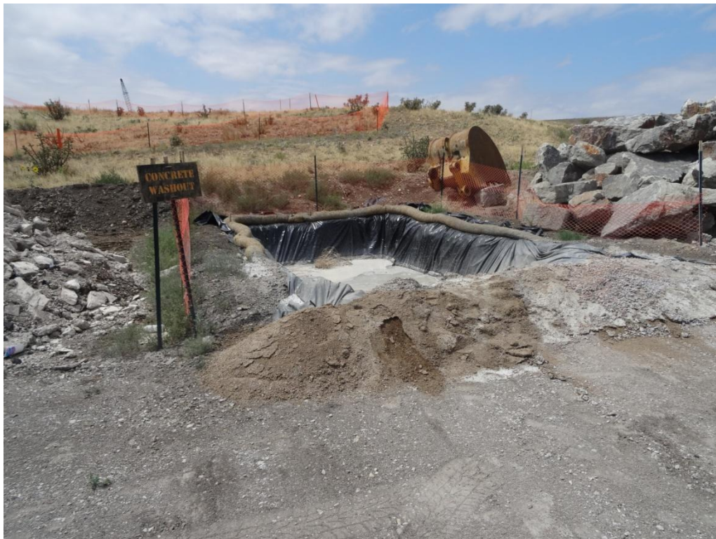
Photograph 11: Concrete washout spilled outside of straw wattle and berm area
