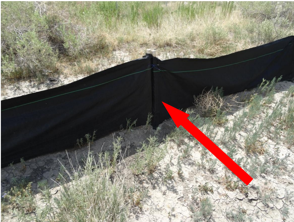
Photograph 8: Silt fence does not adjoin in accordance with good engineering, hydrologic, and pollution control practices to prevent bypass of sediment and debris
