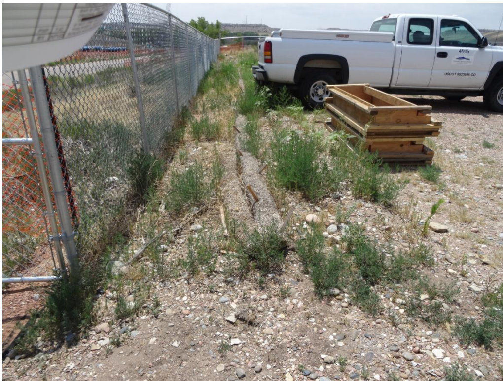
Photograph 1: Straw wattle not installed according to spec and does not facilitate containment of stormwater
