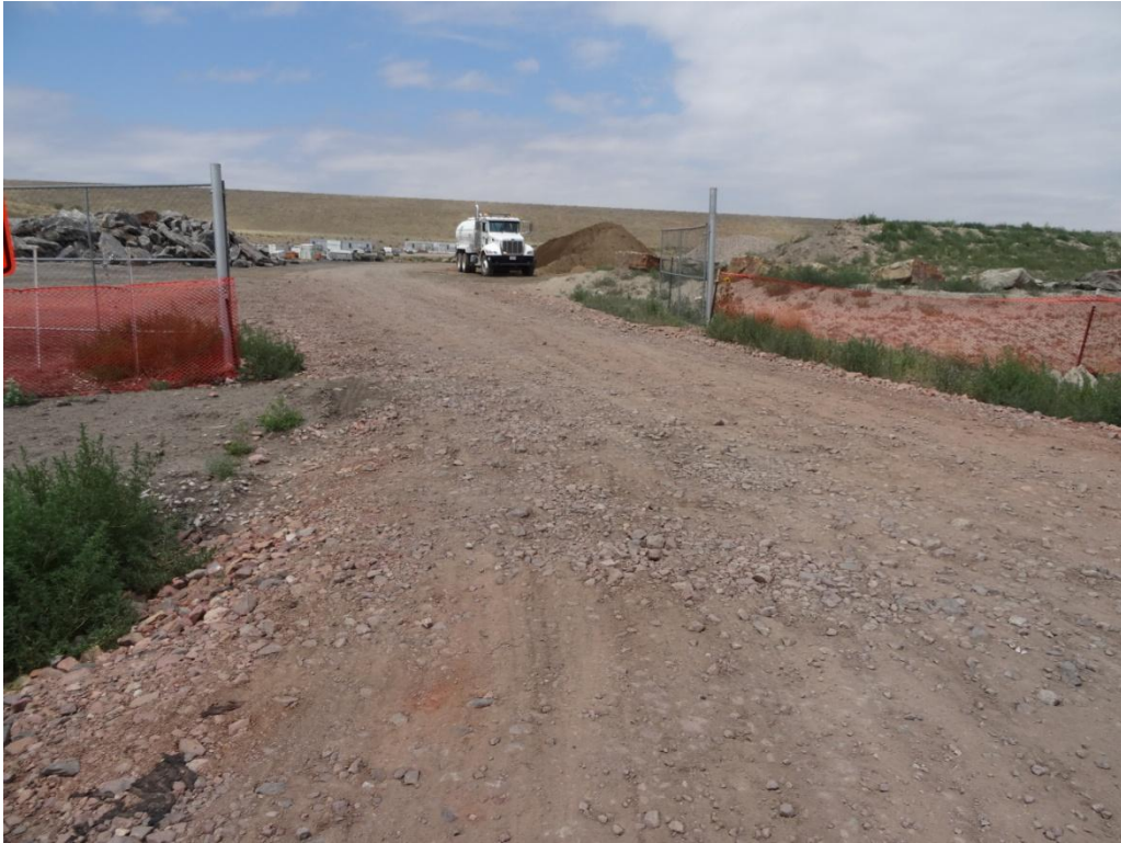
Photograph 7: Vehicle tracking pad into eastern construction area in need of maintenance and additional rock
