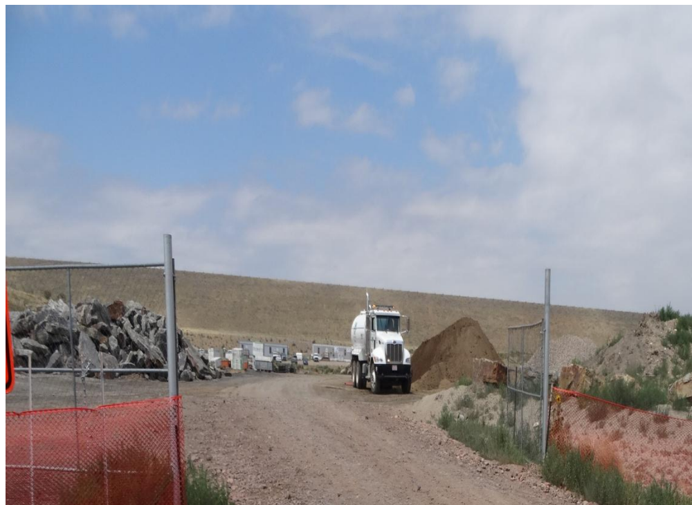
Photograph 5: Stockpiles in the eastern construction staging area without control measures
