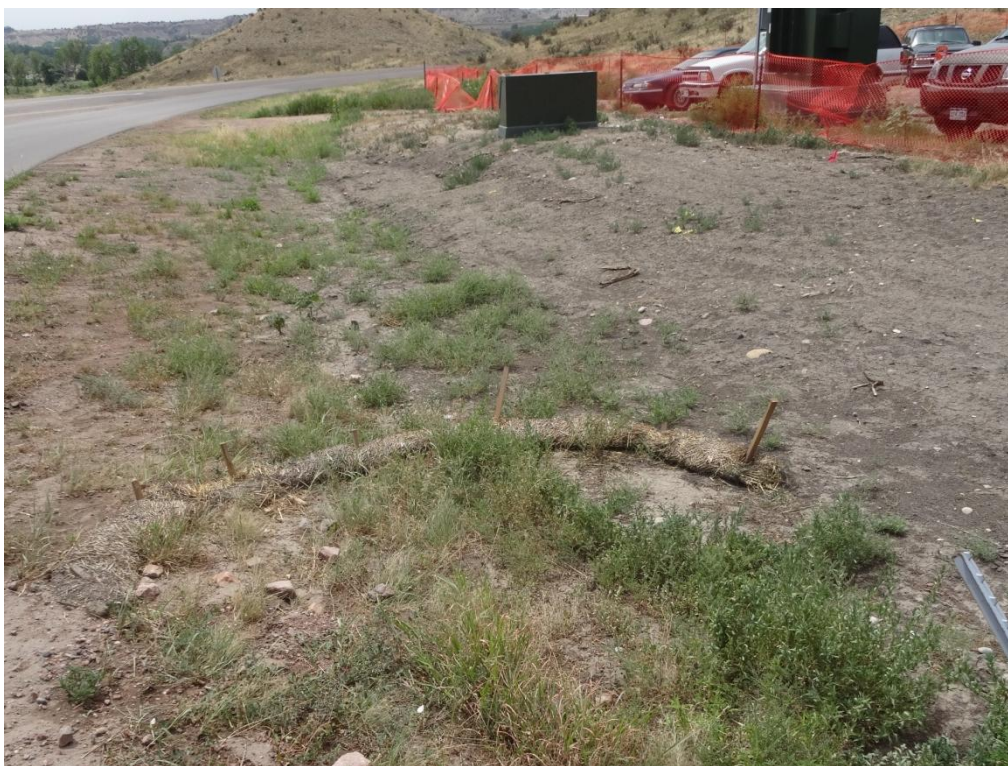
Photograph 9: Straw wattle has holes and tears and is in need of maintenance
