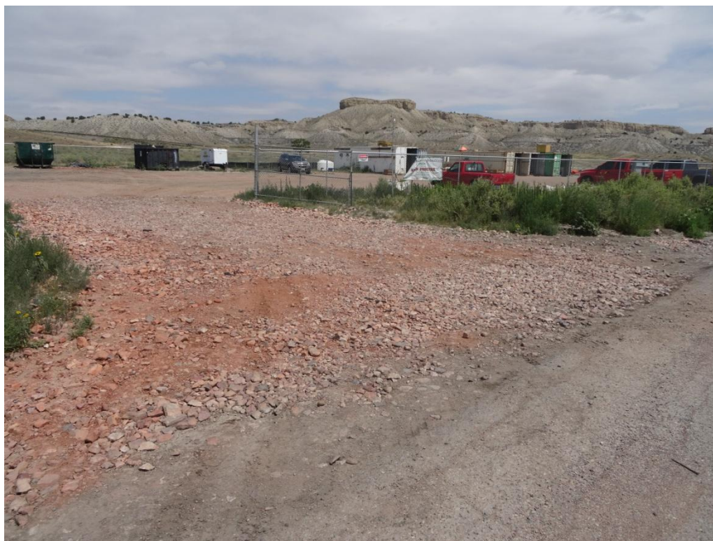
Photograph 6: Vehicle tracking pad into the northern construction staging area in need of maintenance
