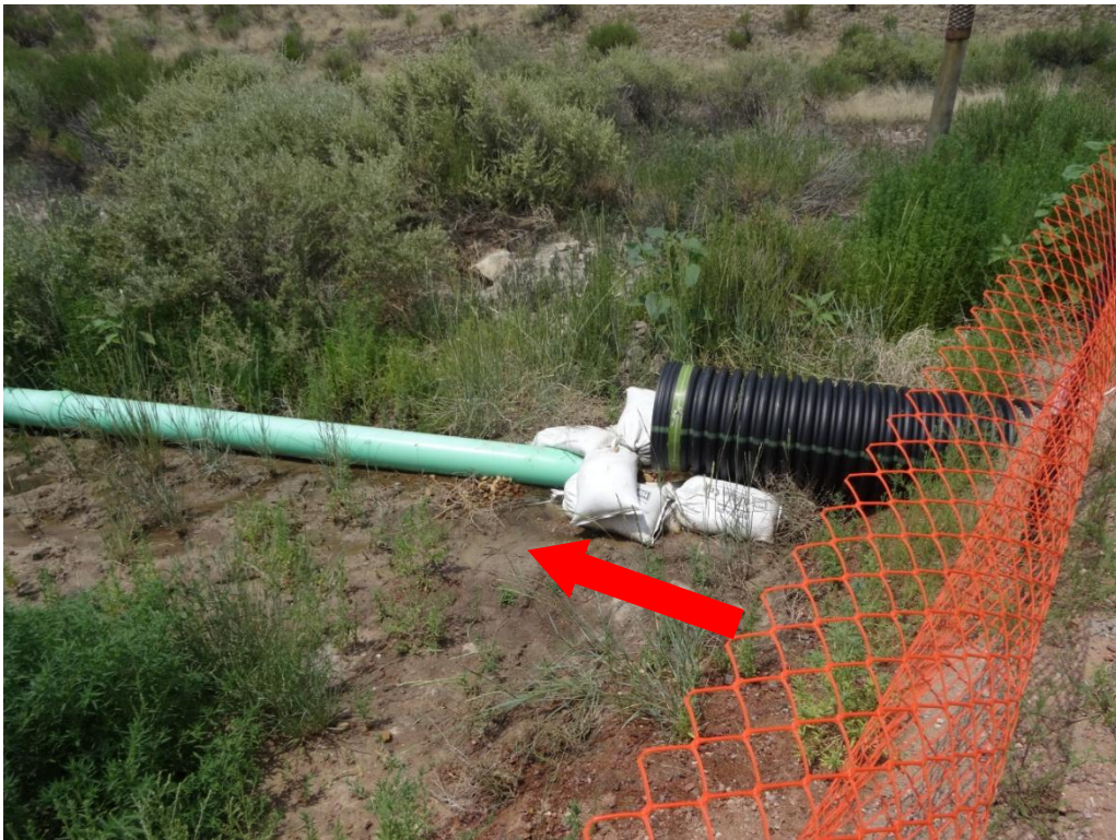
Photograph 2: Arrow points to groundwater dewatering bypassing the piped system to the designated outfall; water is running onto site and into construction activities.
