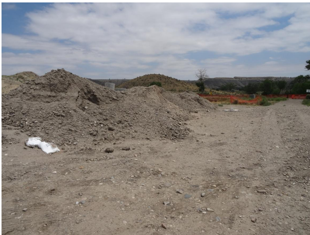
Photograph 3: Stockpiles from excavation on southern side of site with no control measures
