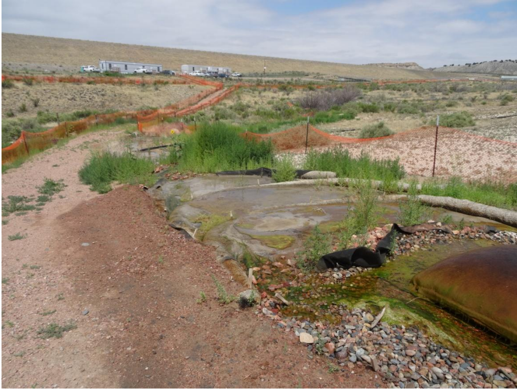
Photograph 1: Sediment built up on straw wattles and filter bag, in need of maintenance.
