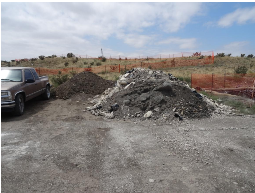
Photograph 2: Stockpiled materials in the eastern construction staging area with no control measures
