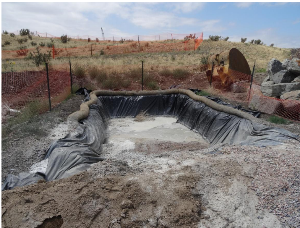
Photograph 10: Straw wattle berm not staked down according to specification
