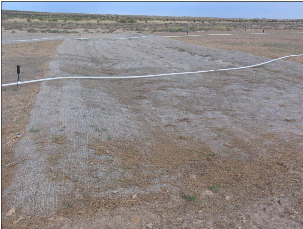
Small drainage with erosion control netting near Southern end of the S3 section of the SDS pipeline. July 24, 2013.
