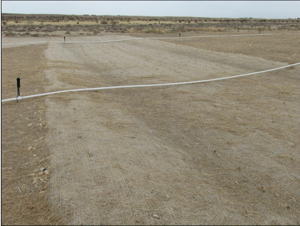
Small drainage with erosion control netting near Southern end of the S3 section of the SDS pipeline. April 30, 2013.
