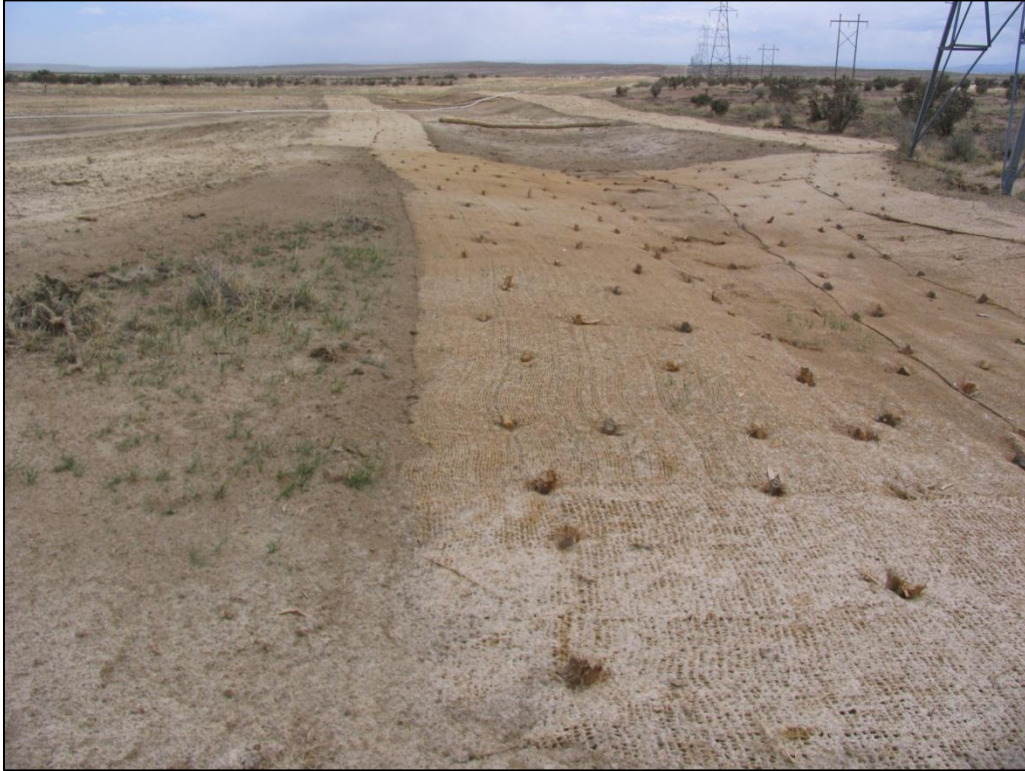
2014 Erosion Control fabric installation along northern Portion of the S3 section of the SDS pipeline South of Antelope Road (Looking Southeast). April 30, 2014.
