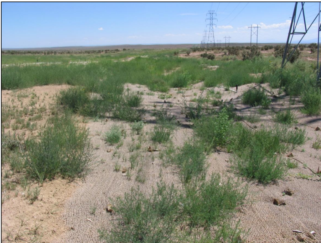
2014 Erosion Control fabric installation along northern Portion of the S3 section of the SDS pipeline South of Antelope Road (Looking Southeast). July 22, 2014.
