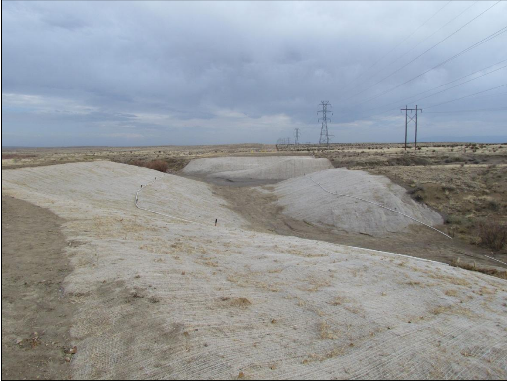
Erosion control netting installed at the Steel Hollow Crossing point along the S3 section of the SDS pipeline (looking southeast). April 30, 2013.
