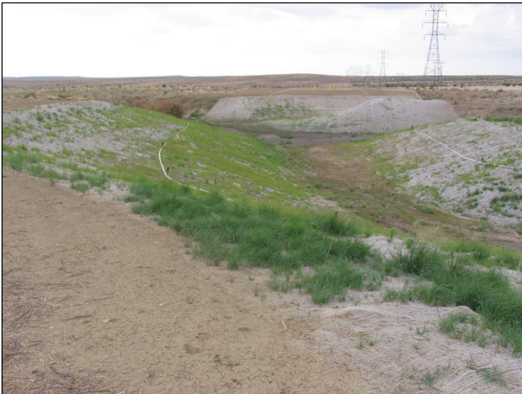
Erosion control netting installed at the Steel Hollow Crossing point along the S3 section of the SDS pipeline (looking southeast). July 24, 2013.
