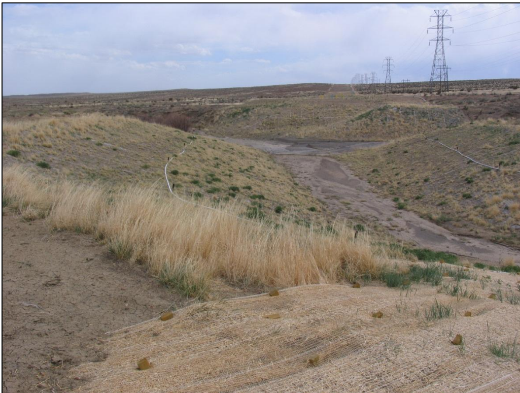
Vegetation growth on erosion control netting installed at the Steel Hollow Crossing point along the S3 section of the SDS pipeline (looking southeast). April 30, 2014.
