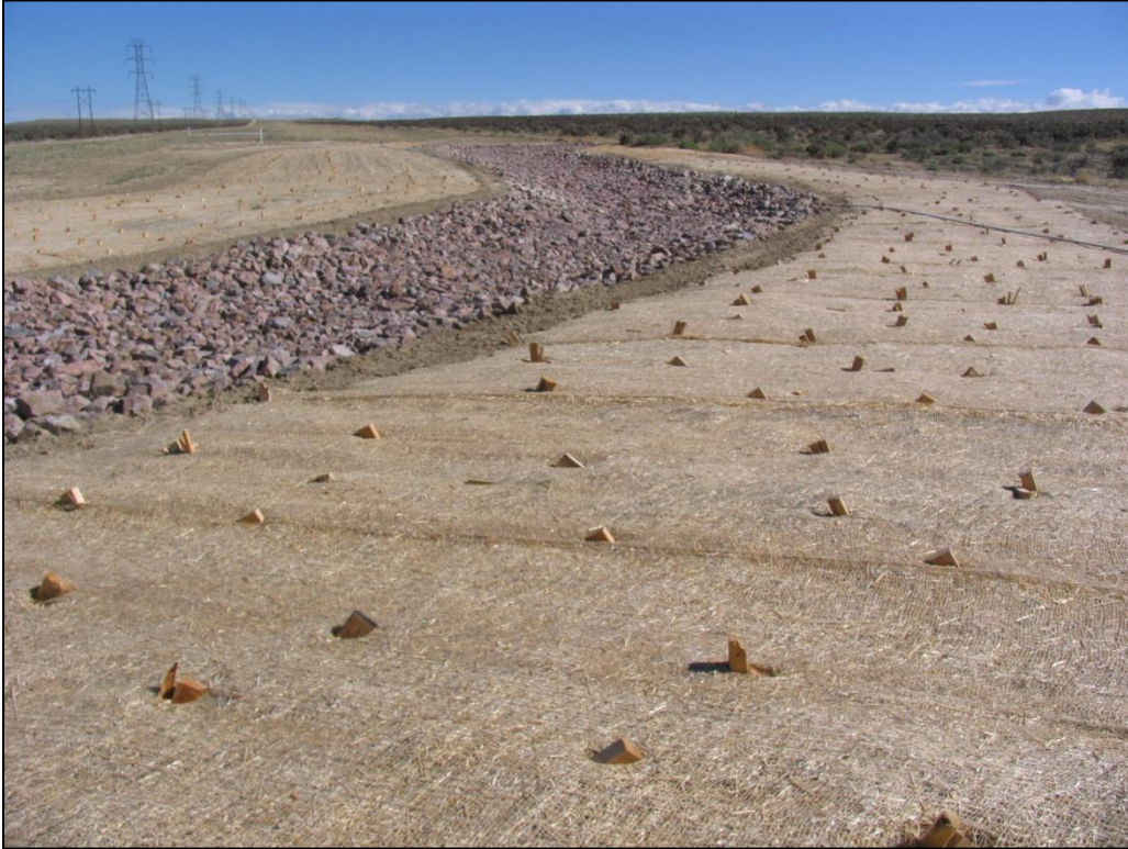
Rip-Rap drainage channel installed in early 2014 in Southern Part of S3 section of the SDS pipeline. April 29, 2014.
