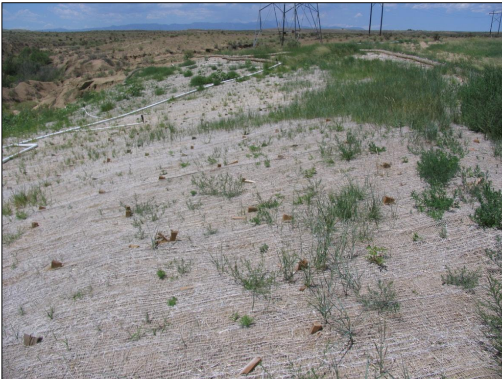
Vegetation growth on erosion control netting installed in 2014 at the Steel Hollow Crossing point along the S3 section of the SDS pipeline (looking northwest). July 22, 2014.
