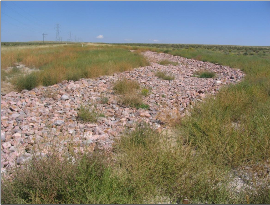
Rip-Rap drainage channel installed in early 2014 in Southern Part of S3 section of the SDS pipeline. September 2, 2014.
