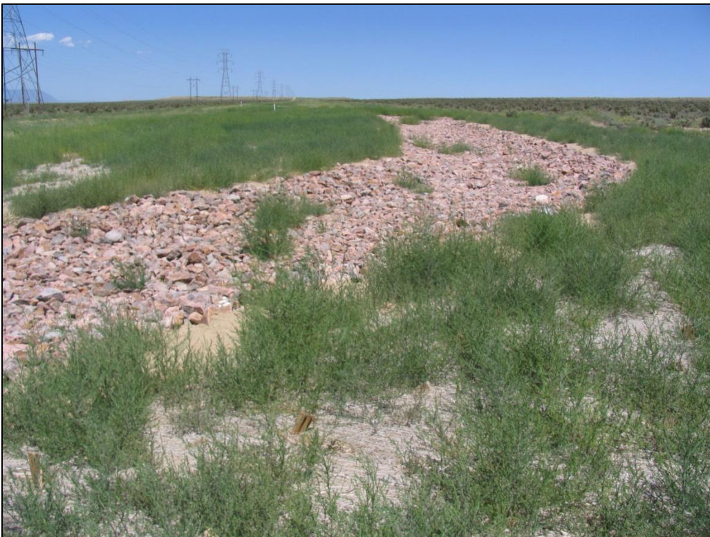
Rip-Rap drainage channel installed in early 2014 in Southern Part of S3 section of the SDS pipeline. July 22, 2014.
