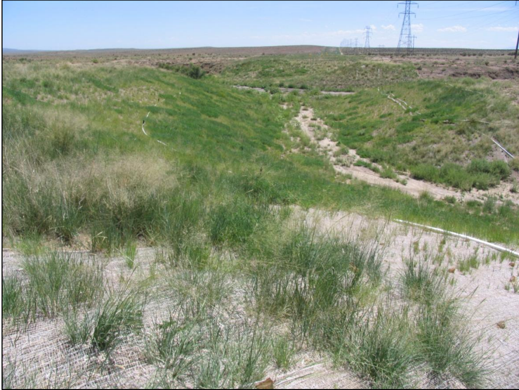
Vegetation growth on erosion control netting installed at the Steel Hollow Crossing point along the S3 section of the SDS pipeline (looking southeast). July 22, 2014.
