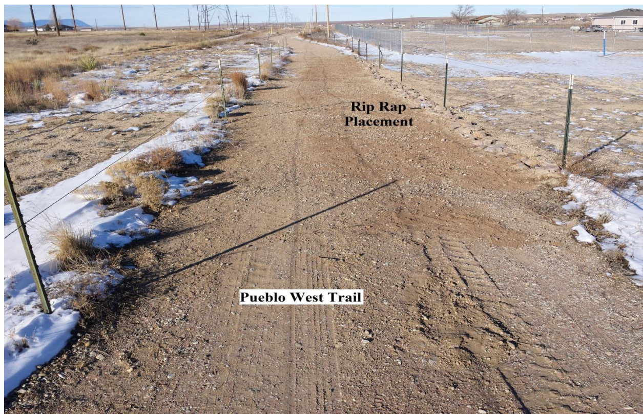
Rip-Rap placement along downstream side of trail for erosion control. 12-15-2015
