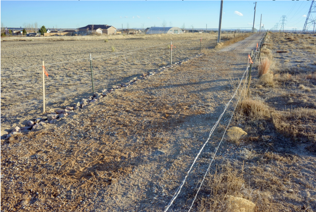
View looking southeast at the former location of two rills across the Pueblo West Metropolitan District recreation trail following restoration and rock installation.
