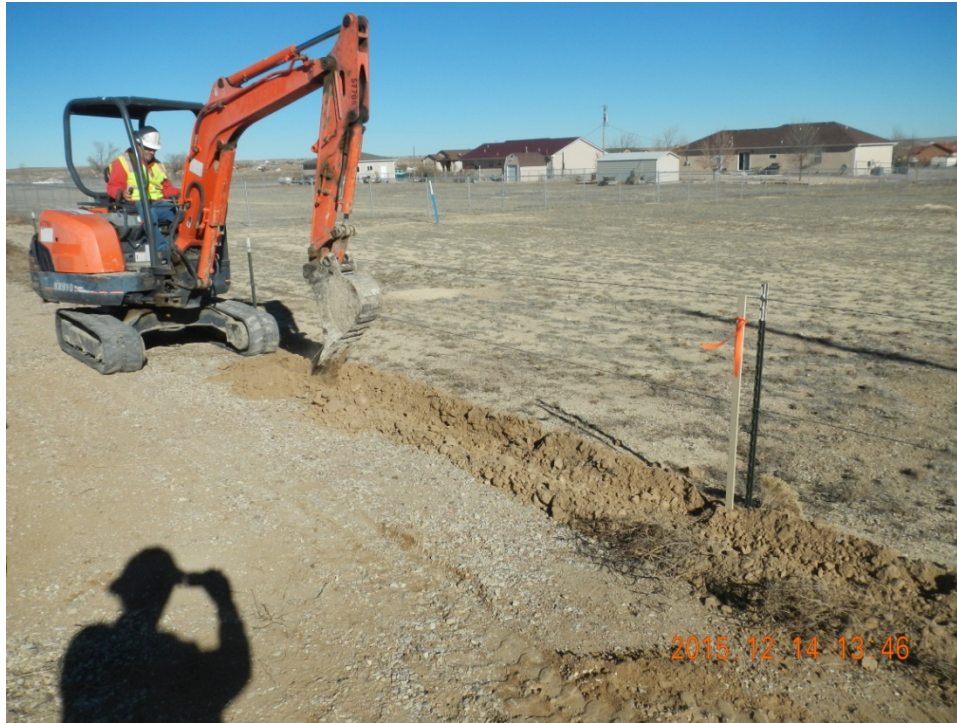
View looking northeast during the shallow trenching activities along the eastern boundary of the recreational trail prior to rock installation.
