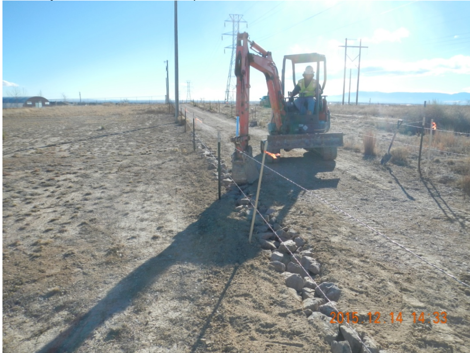
View looking south at the rock placement and compaction conducted during the rock installation activities along the eastern boundary of the recreation trail.
