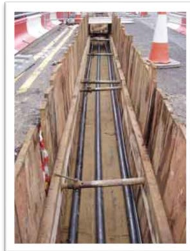
Figure 7-2 Direct Buried Installation- Urban
