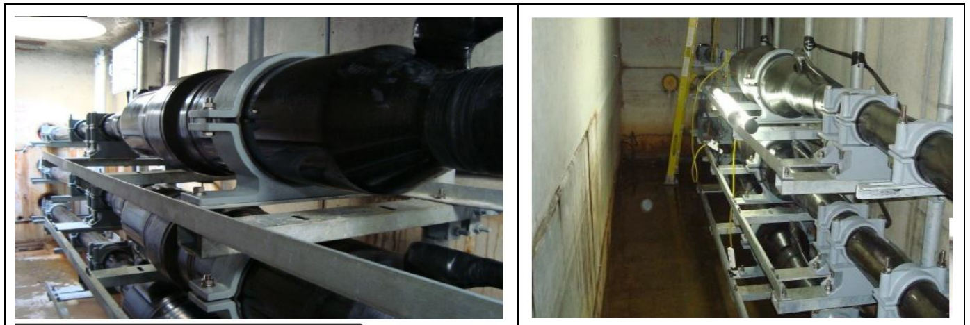
Figure 9-3 Actual Installation of Cables and Joints in Straight through Arrangement
