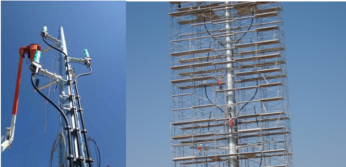
Figure 13-5 Cable Termination Installation on Transition Pole
