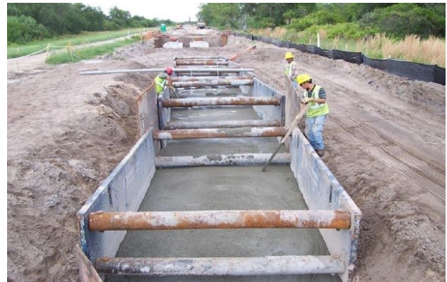
Figure 12-3 Conduit Backfilling
