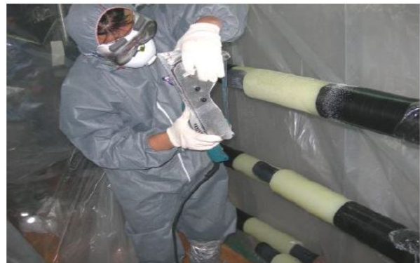
Figure 13-4 Preparing the Cable End
